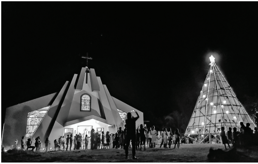
The newly built St. John the Baptist Parish Church on the historic Homonhon Island in Guiuan, Eastern Samar. PHOTO BY FR. CHRISTIAN OFILAN
