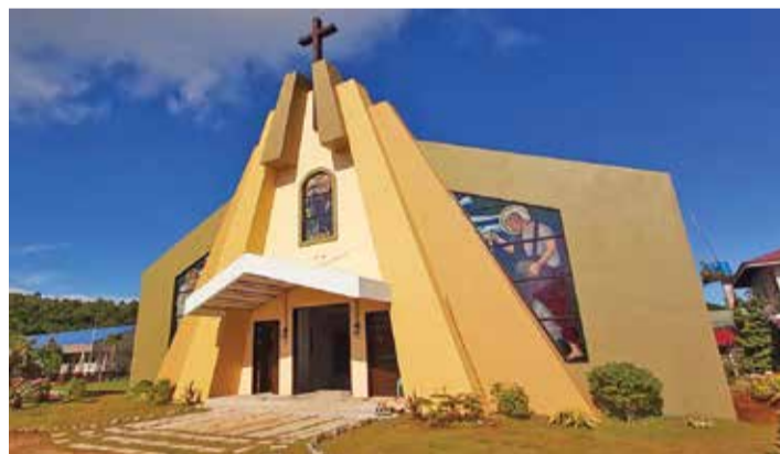
The newly built St. John the Baptist Parish Church on the historic Homonhon Island. CBCPNEWS
